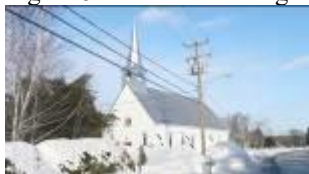
Figure 5.41 St.James Anglican Church
